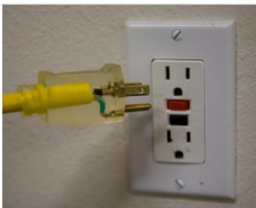
Level 1 Charging - Standard House Outlet
